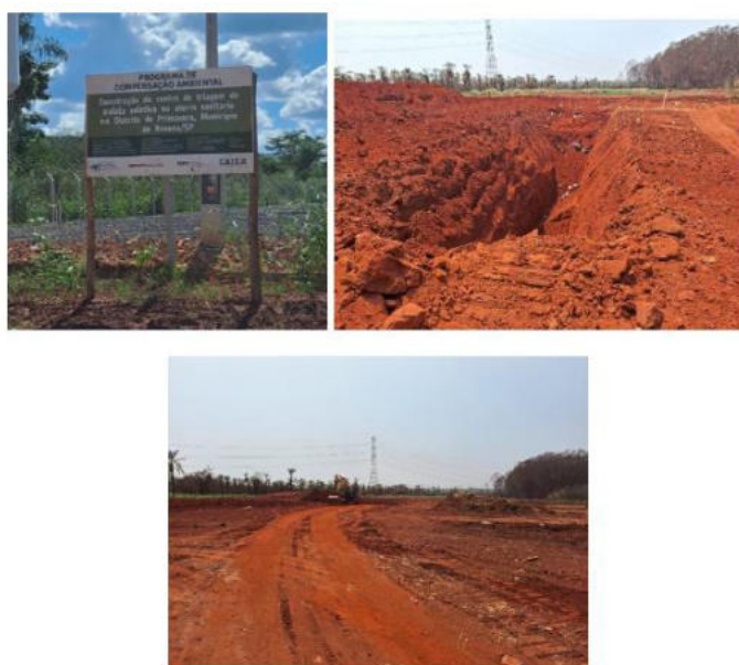
Figure 1. Situation of the Rosana Sanitary Landfill
